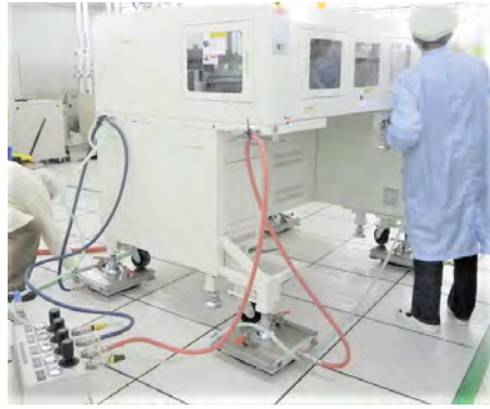
Figure 2. With the machine's wheel placed on the aluminum square housing the air caster, weight is efficiently redistributed, alleviating any issue with floor point loads on raised floors.
