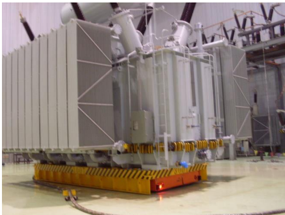
Transformers move safely and efficiently on air.
