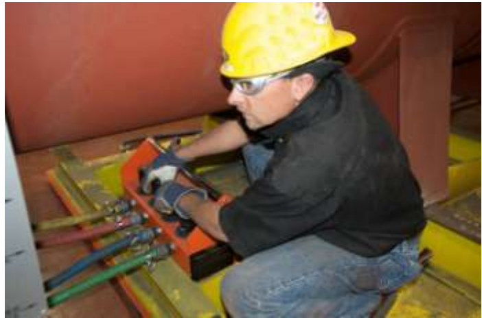
Compressed air Control Box makes it possible for one operator to manipulate the megaton equipment into place.
