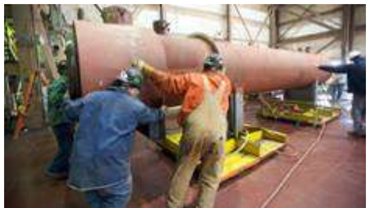
Megaton feedwater heaters glide easily on air casters.
