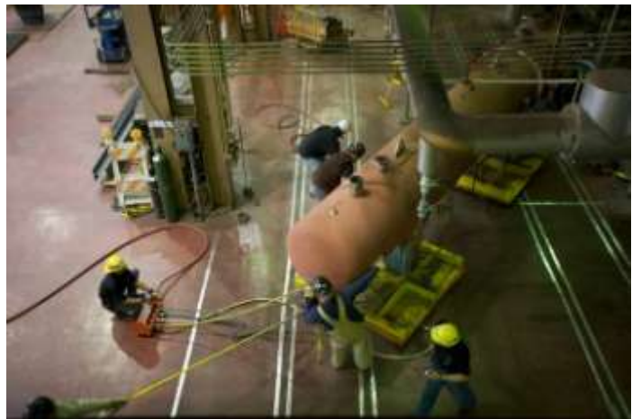
Overhead view of feedwater heater moving into position.
