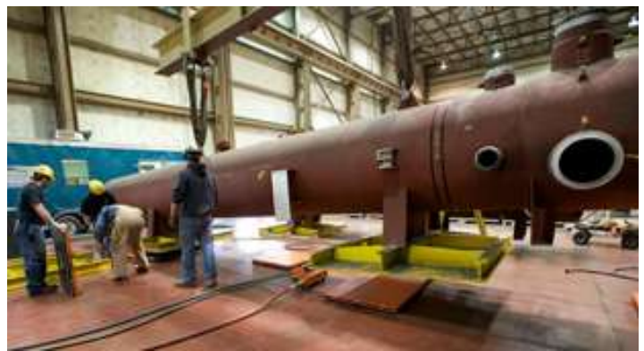
The replacement feedwater heater is placed on air casters.
