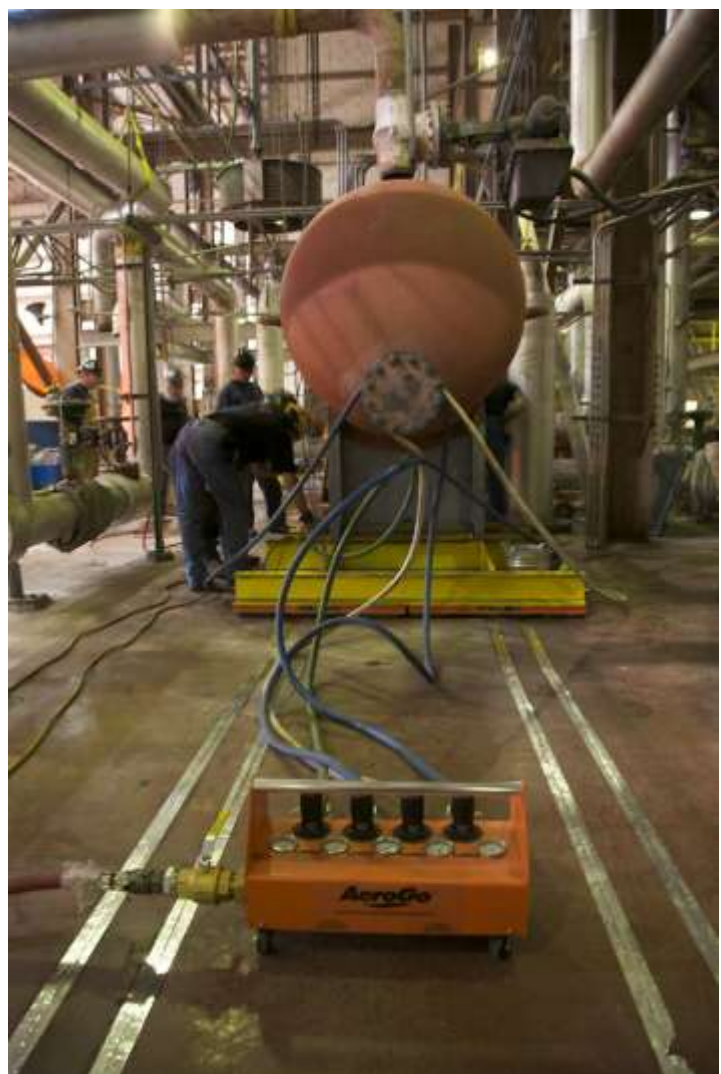
Save plant downtime by days just by utilizing air casters and a control box.
