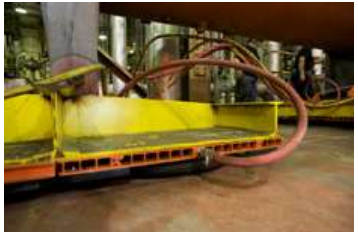
Using on-site compressed air, the air caster lifts the feedwater heater
