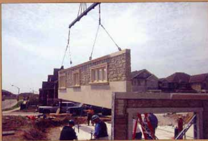
Thermally efficient steel studs combine with thin shell concrete by TMCP Building System to panelize fourteen 5,000 sf homes each day
