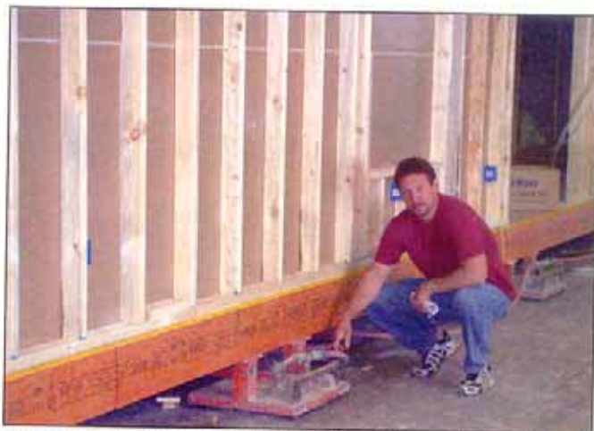
Fink shows one of the AeroGo Aero-Casters at the end of a Load Beam. The Aero-Caster Load Beams make it easy to move modulars in any direction.
