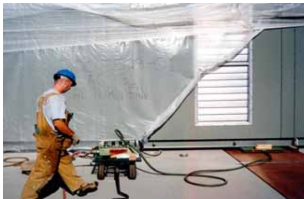
27-inch Aero-Caster Load Module Systems were used with some shimming to compensate for the off-centered load weight.
